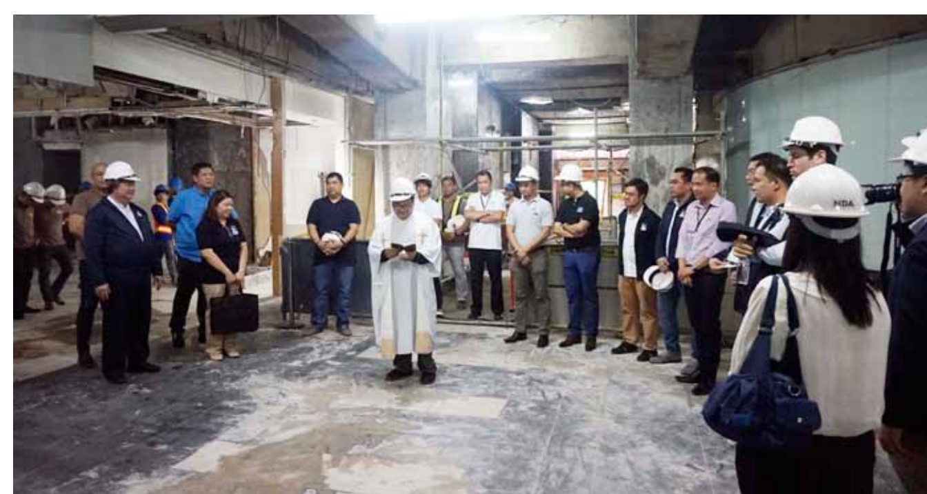
A priest blesses the Insular Life Makati grounds prior to the start of the construction.
